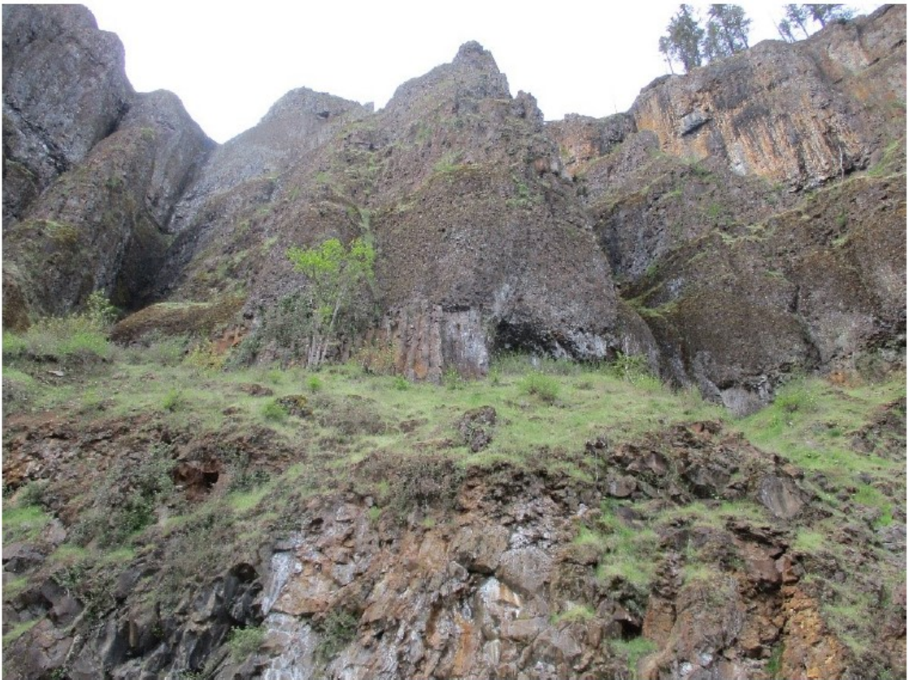
Photo 3 - Big Cliff, May 2023. Note the fault just right of center
